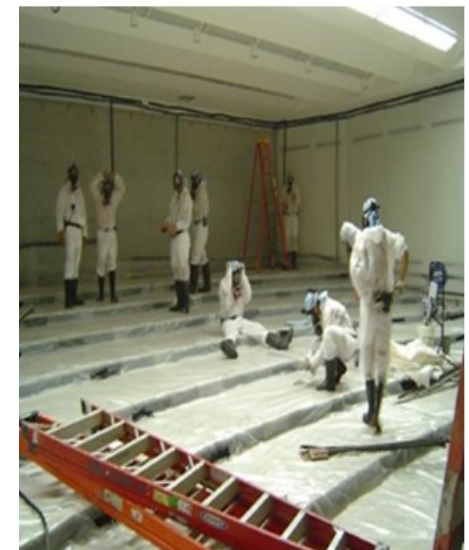
PPE use during asbestos removal
